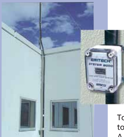
The ERICO ERICORE Downconductor is easily retrofitted to existing structures. Inset: ERICO Lightning Event Counter (LEC IV) installed to register strikes to ERICO SYSTEM 3000.
